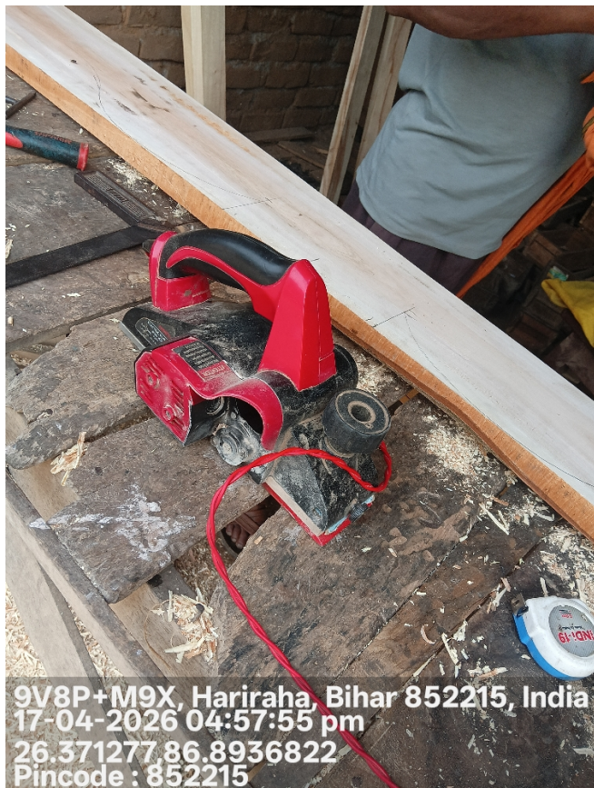
Photo of Machinery Setup
