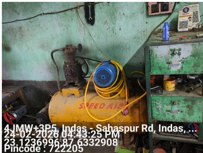
Photo of Machinery Setup
